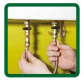
If by mistake the pressure is topped up more than 2 bar then go to the 'how to bleed a radiator' page and follow the steps. You can use this method to take the excess water out of the heating system until the pressure returns back to between 1 and 1.5 bar.
